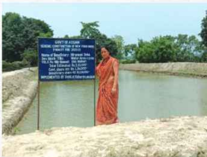
New pond construction under PMMSY
